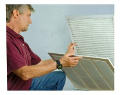
system, the system can't perform well without one. Dust and grime accumulate on critical parts, like the evaporator coil, causing unnecessary wear and tear.
